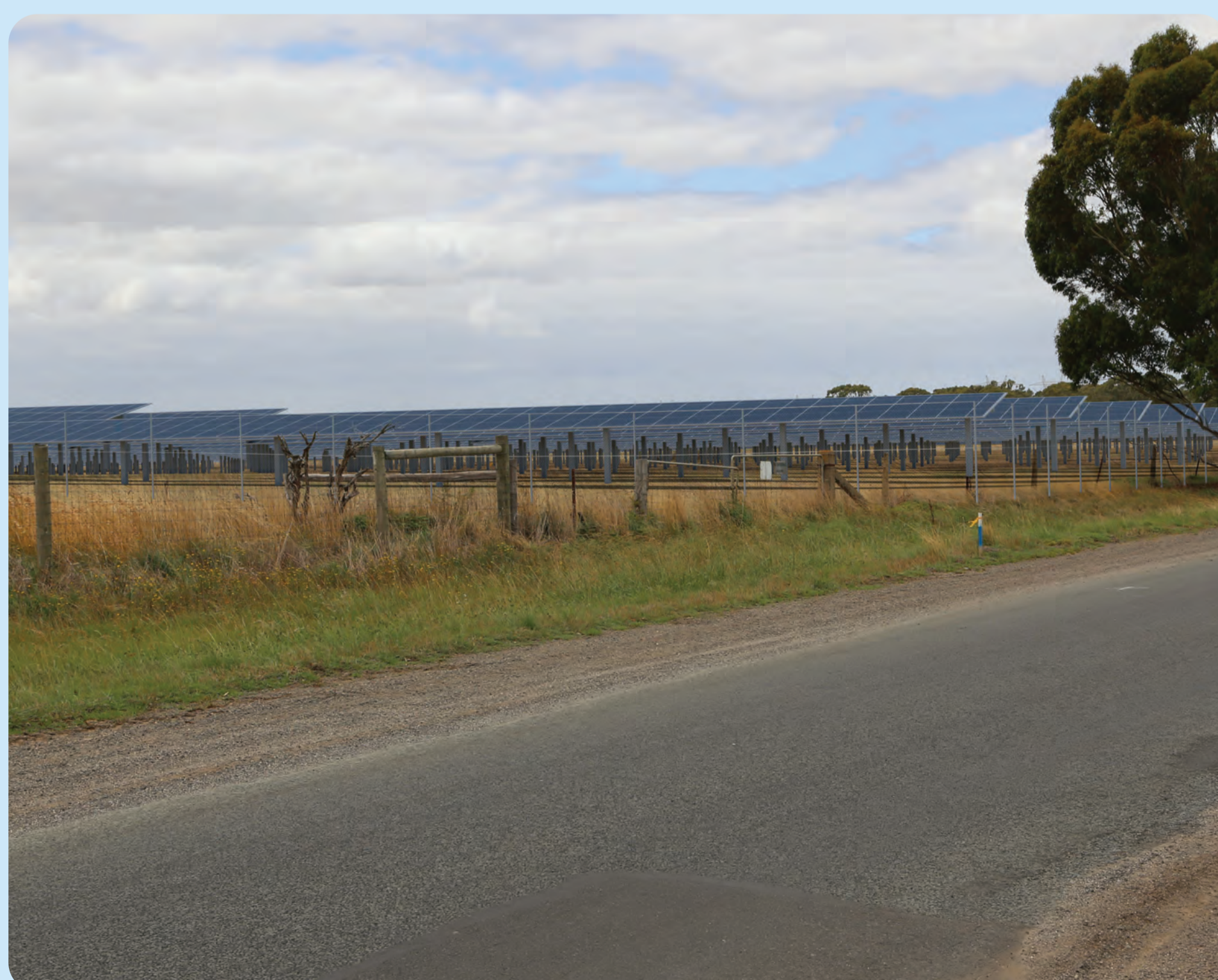
VP 3: Looking ENE at the proposed solar farm from Little River-Ripley Road
