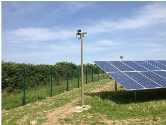
CCTV camera in centre of above photo.
