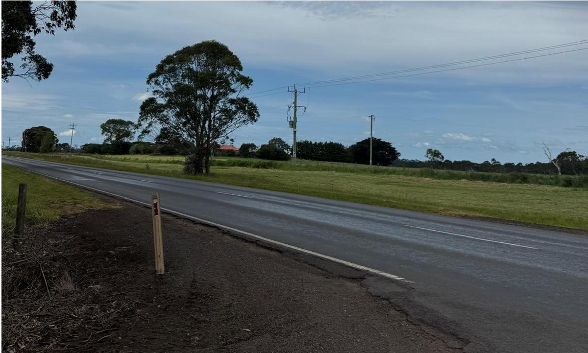
Figure 4. Connection into the 66k V distribution network located along Cobden-Warrnambool Road. Source: DTP Officer
