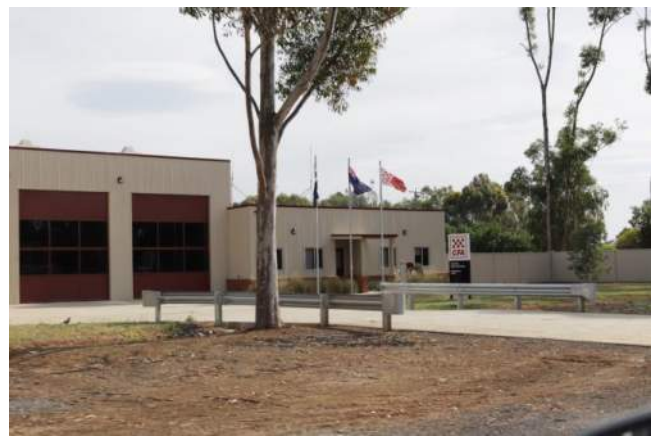
Photo 6.2 View from O'Reilly Road, Tatura facing north showing Tatura Fire Station
