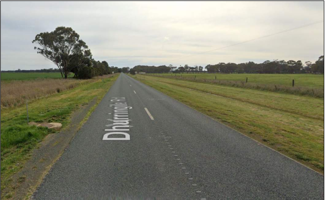
Figure 4 Dhurringile Road facing north adjacent to subject site
