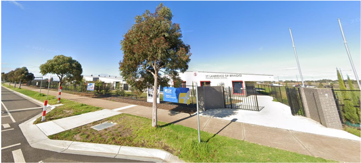
Figure 12 Existing primary school entrance as viewed from Waterway Boulevard (April 2023)
