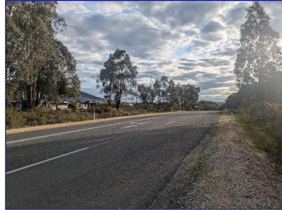
Figure 7: John Schubert Drive - View West
