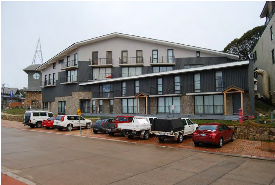
Figure 1: View of Molonys Apartments from (north) New Summit Road- showing existing road, footpath, retaining wall, hydrant and grassed areas. Not to be impacted by construction activities + grass made good if trampled.
