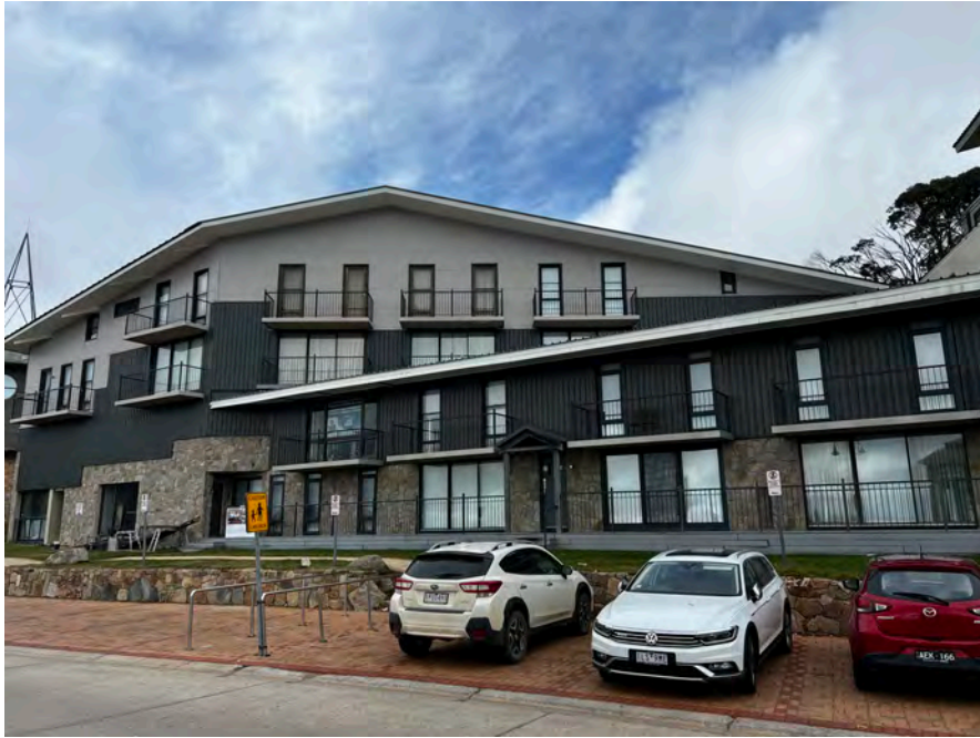
Figure 3.3: Subject building showing existing roofing and balconies to be replaced
