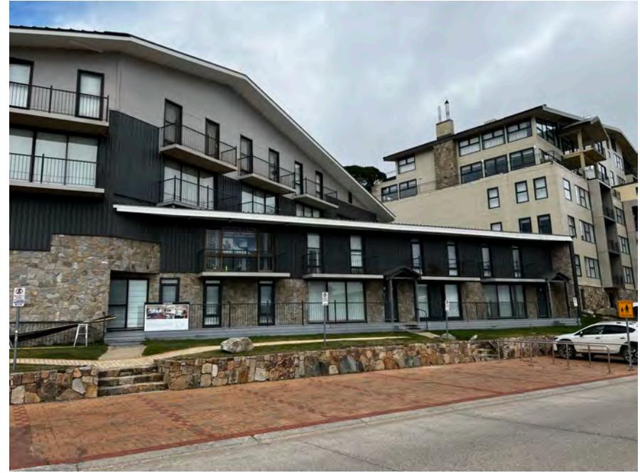
Figure 3.4 Subject building showing existing roofing and balconies to be replaced
