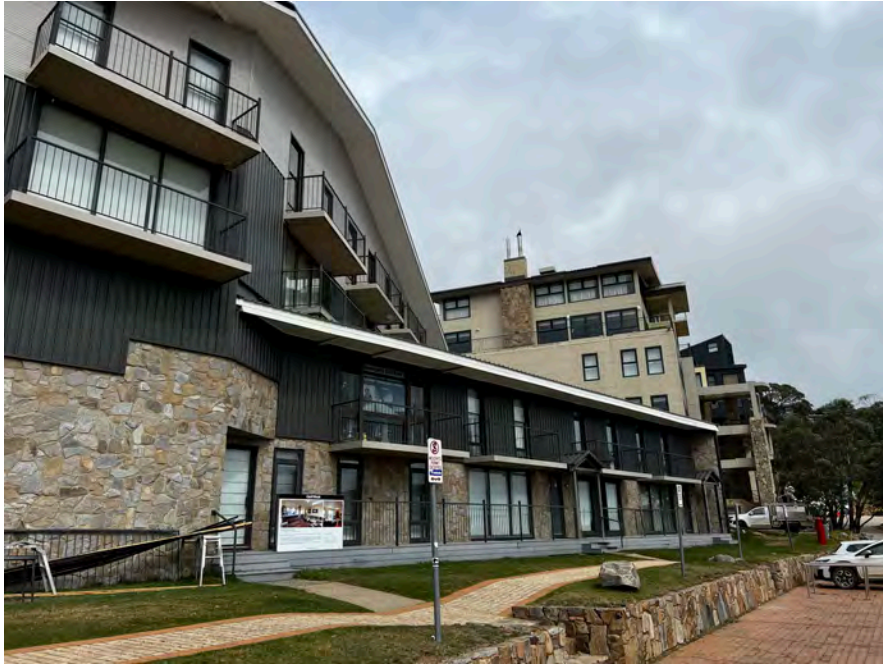
Figure 3.5: Subject building showing exiting roofing and balconies to be replaced
