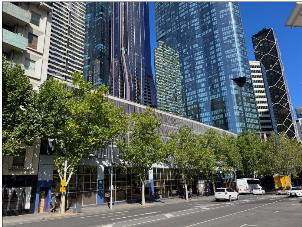
Figure 10: Subject site - western elevation (Queen Street) (Source: Site Visit - 12 February 2026)
