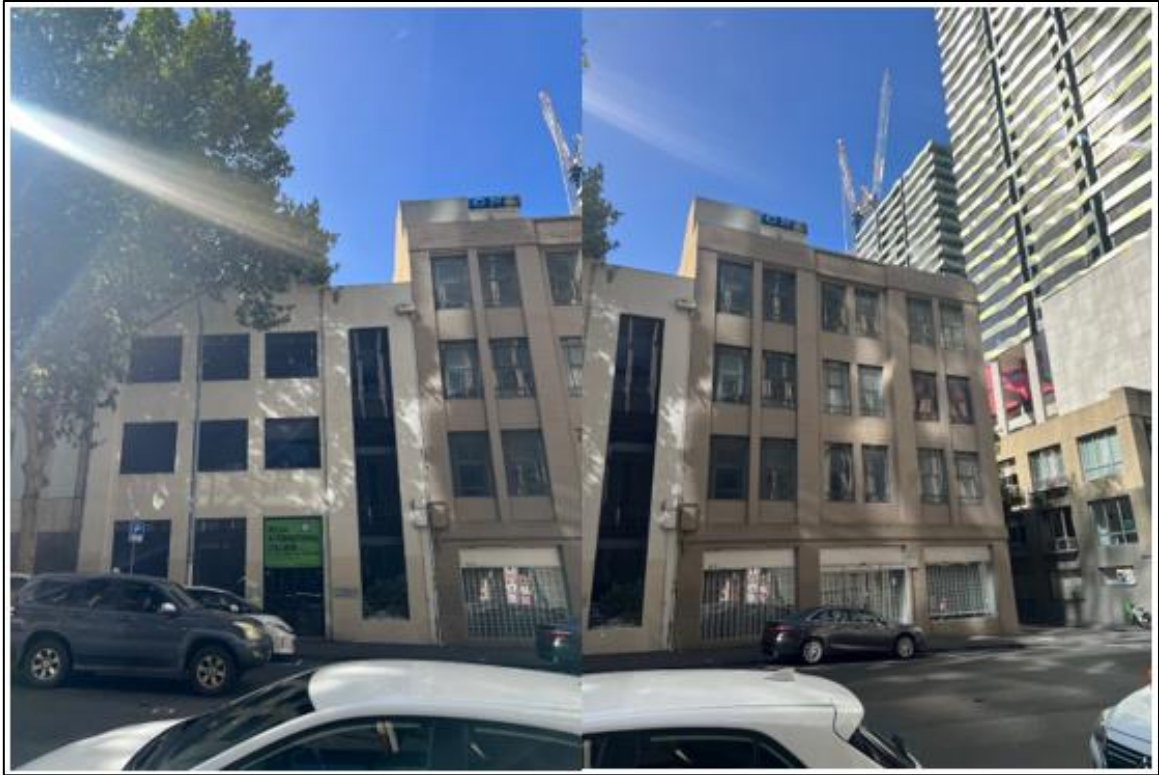
Figure 14: 150-154 A'Beckett Street (left) and 144-148 A'Beckett Street (right) (Source: Site Visit - 12 February 2026)
