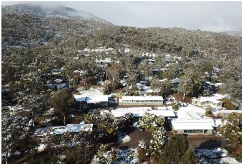
Figure 8: School buildings (source Geelong Grammar)
