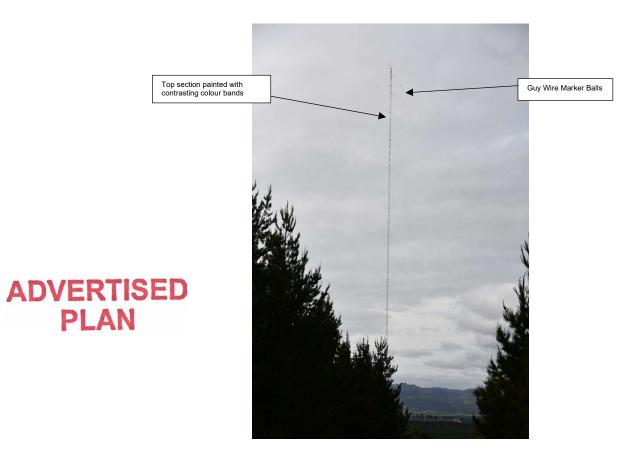
Figure 8 – A Meteorological Monitoring Mast in the DWF
