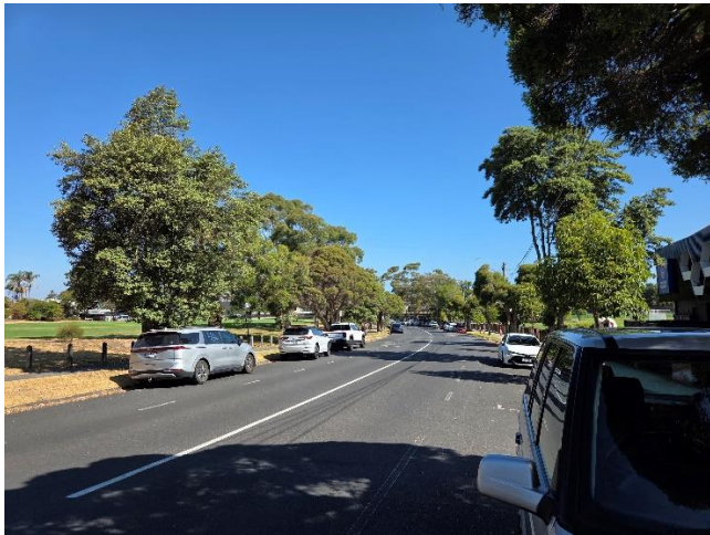
Figure 22 Outer Crescent looking south from the area of works
