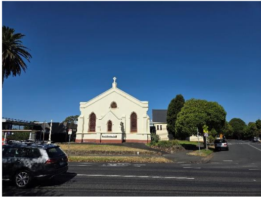
Figure 14 Girrawheen Chapel from New Street
