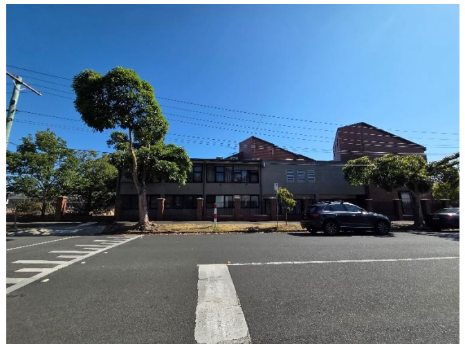
Figure 19 Existing northern elevation to Allee Street
