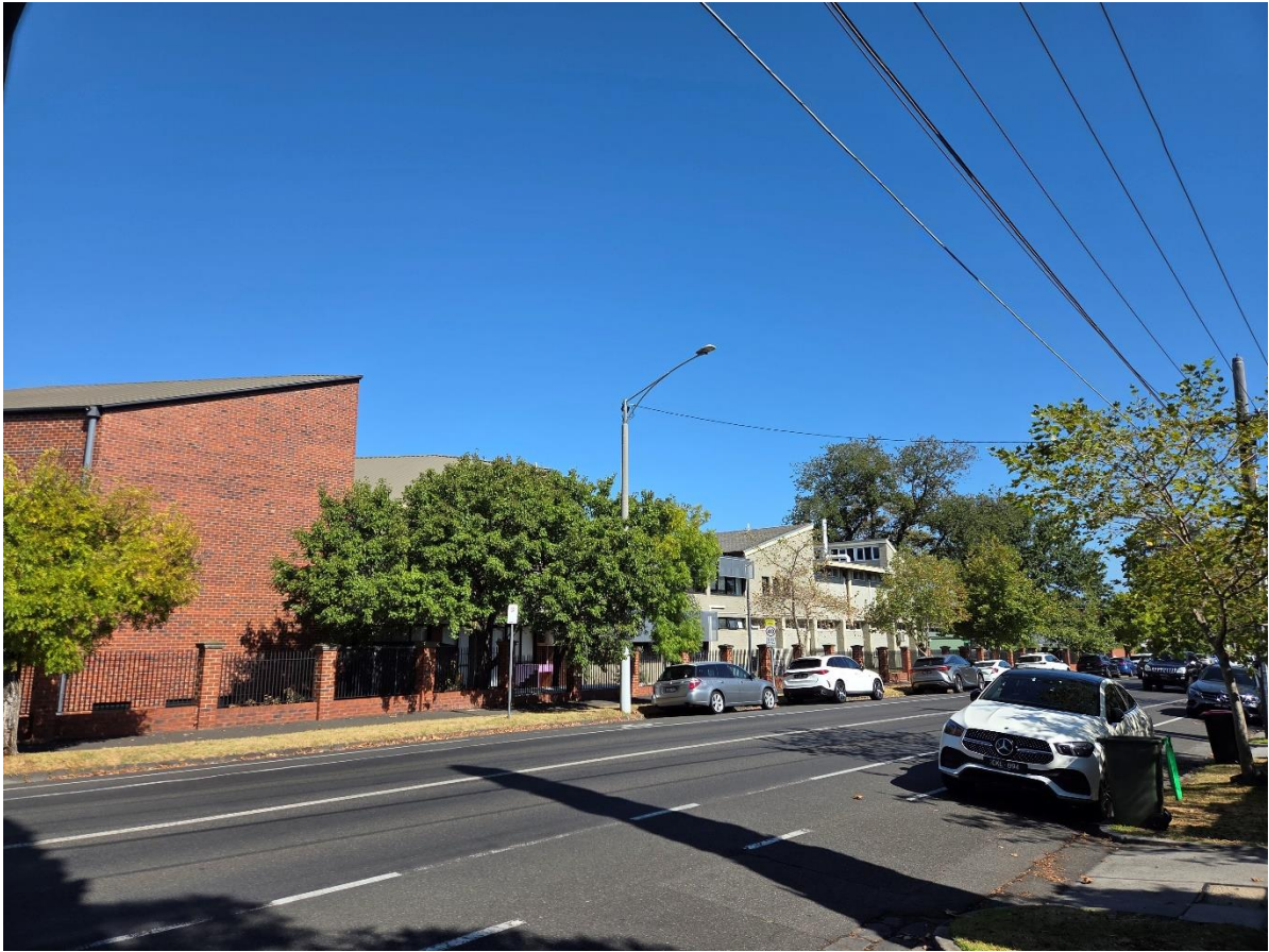
Figure 12 Area of works looking ESE from North Road (existing elevation)
