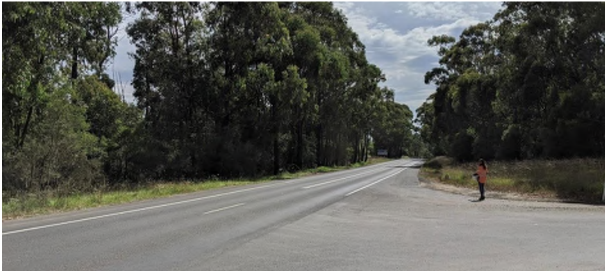
Figure 7 Creamery Road – priority intersection with Strzelecki Highway (Source: AECOM photo taken 19/03/2020)
