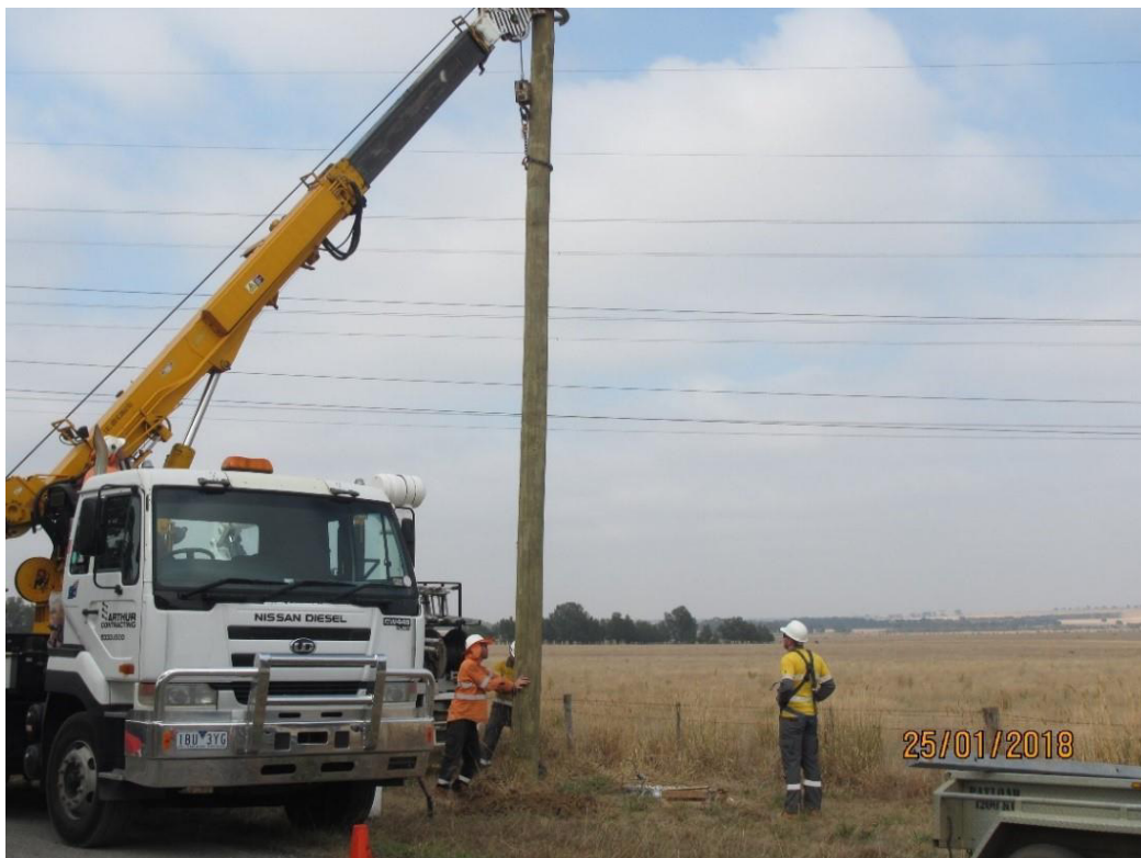
Figure 4: Example of pole being installed via truck crane
