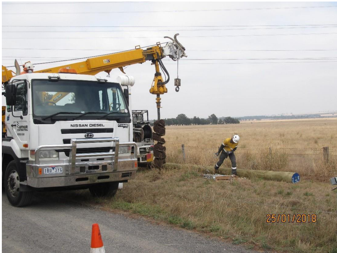
Figure 2: Example of a hole being augured via arm from truck (note in this example the roadside vegetation was deemed to be non-native, hence the truck parking slightly on the verge and the other truck in the background)
