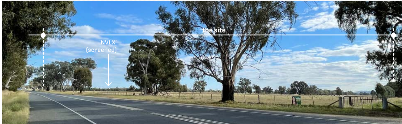
View to the site.
