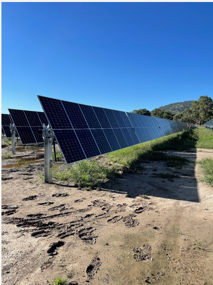
Figure 9 – Example of a typical single axis tracker system with PV modules mounted in single panel portrait orientation (1P configuration)
