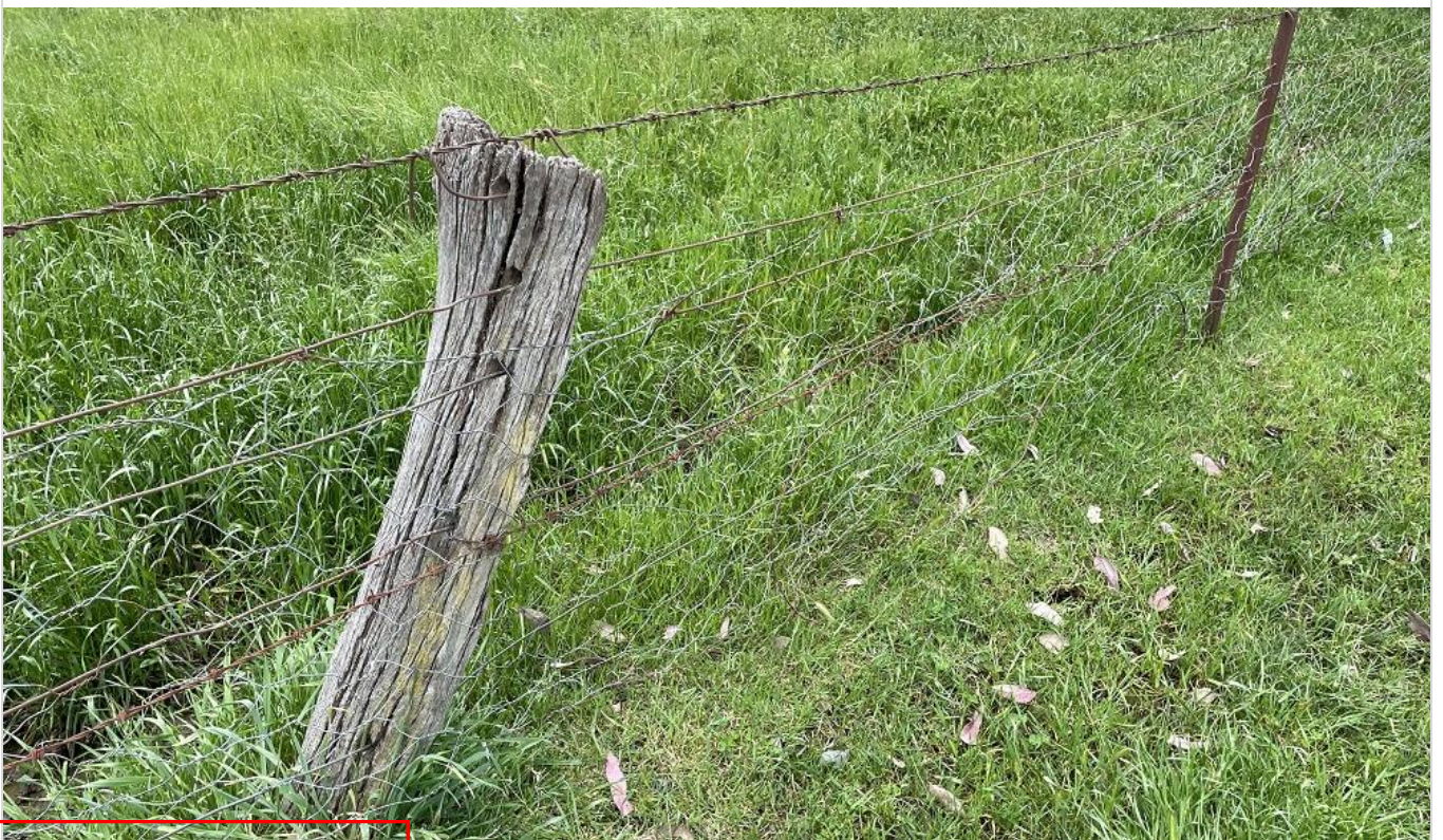
Photo 4: A section of the internal fencing which is nearing the end of its useful life. Fencing along the northern and eastern boundary with adjoining paddocks will likely require replacement to avoid livestock straying into the solar energy facility.
