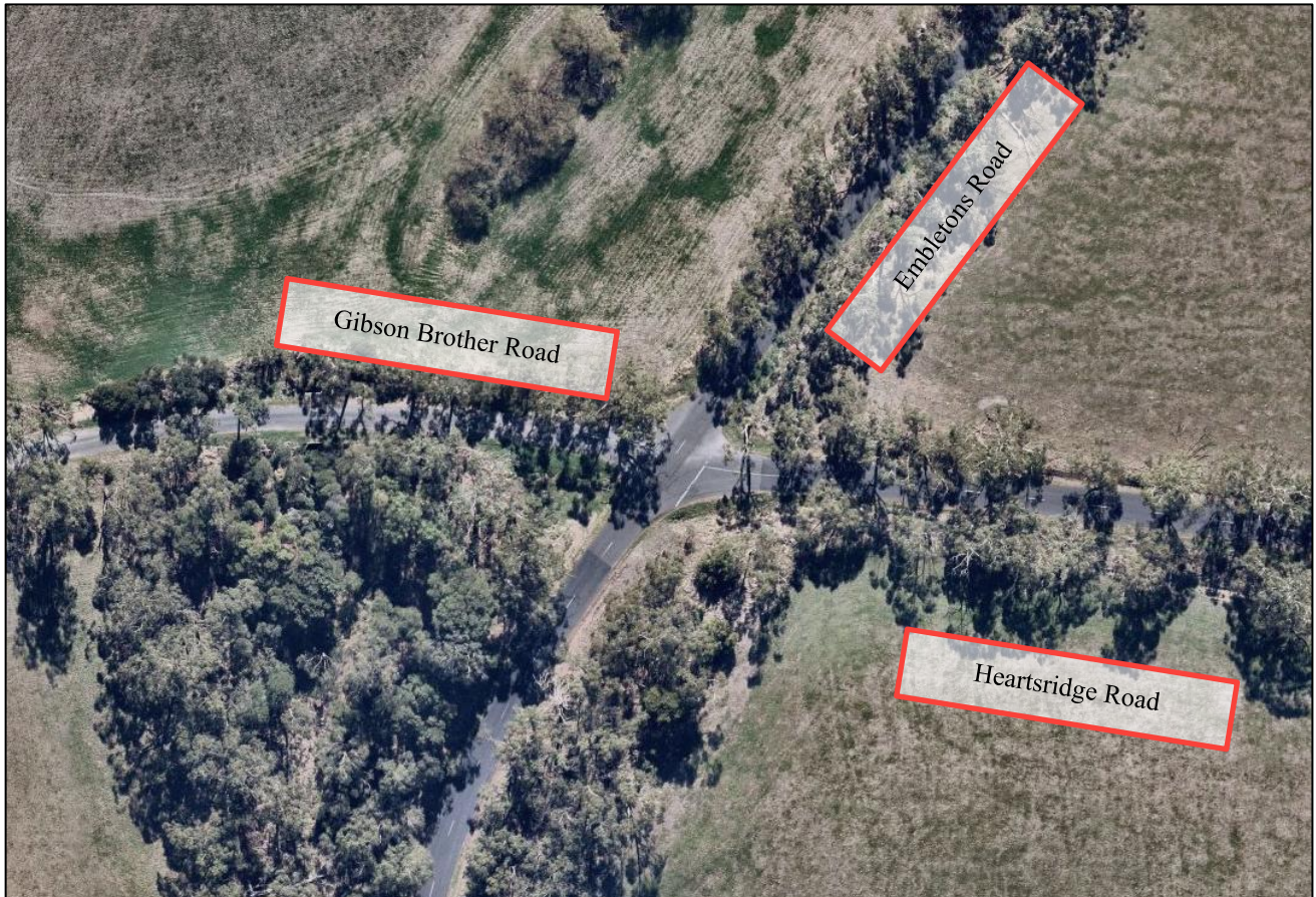
Figure 2-8 Embletons Road / Heartsridge Road
