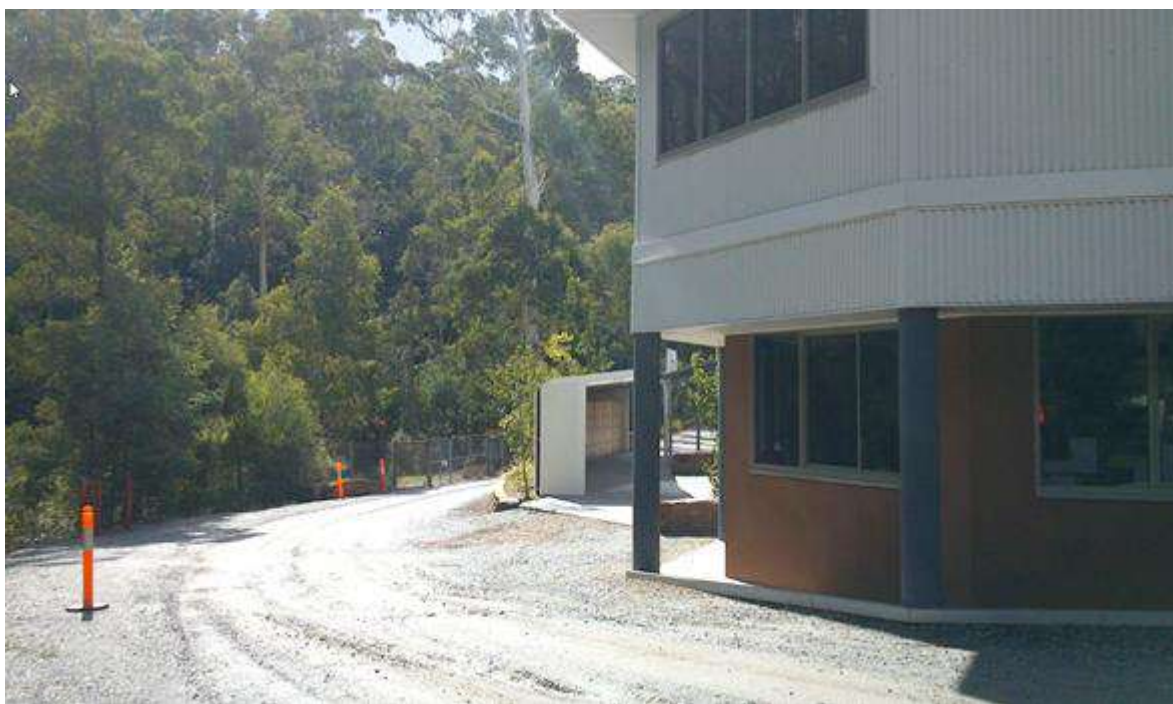
Photograph 5: existing fire access track
