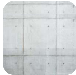
OFF FORM CONCRETE
