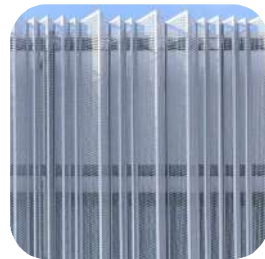
PERFORATED METAL CLADDING LIGHT COLOUR
