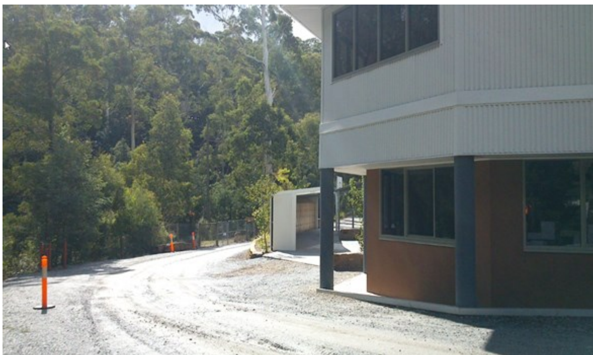
Photograph 5: existing fire access track
