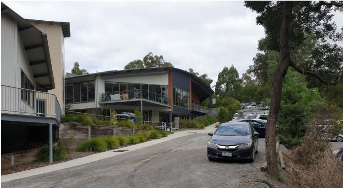
Photograph 1: Existing school built form (middle school building), access and carparking
