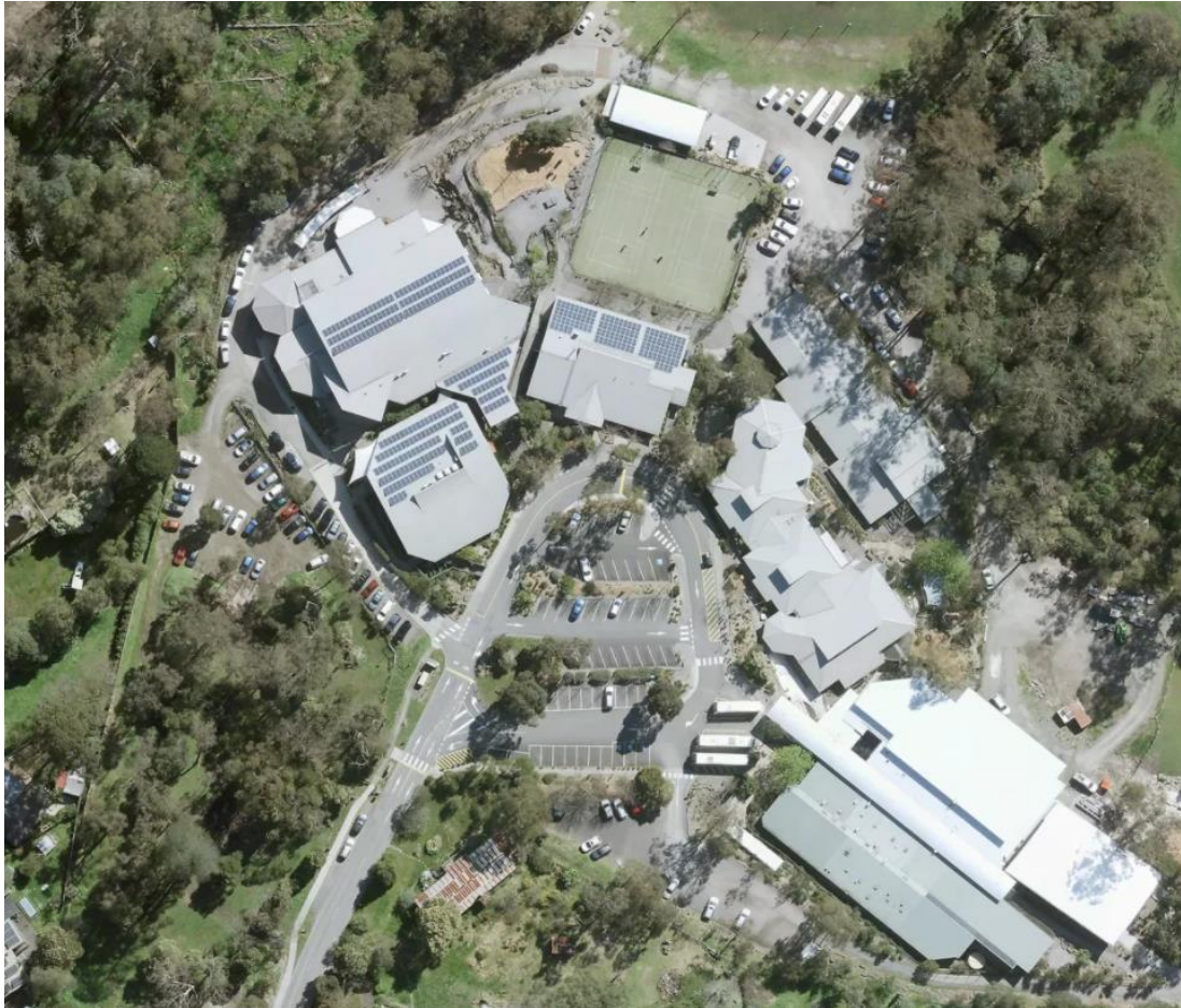
FIGURE 4: EXISTING PARKING ALONG WATTLE VALLEY ROAD AND WITHIN THE SCHOOL PROPERTY
