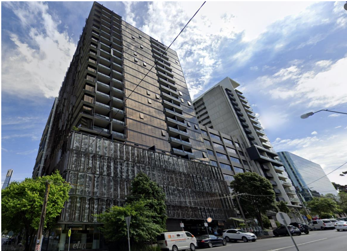
Figure 5: Built form to the north of the subject site
