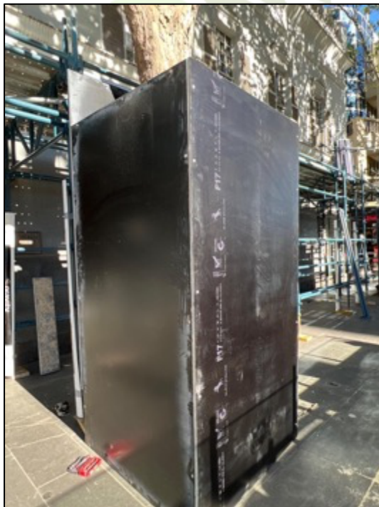
Figure 2. Example of hoarding
