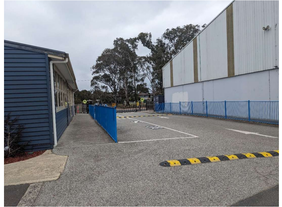
8. Facing south along exit driveway, leading to Breanne Place.
