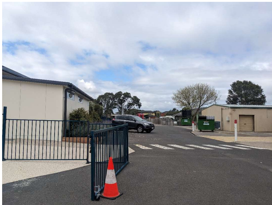
9. Facing east towards maintenance building.
