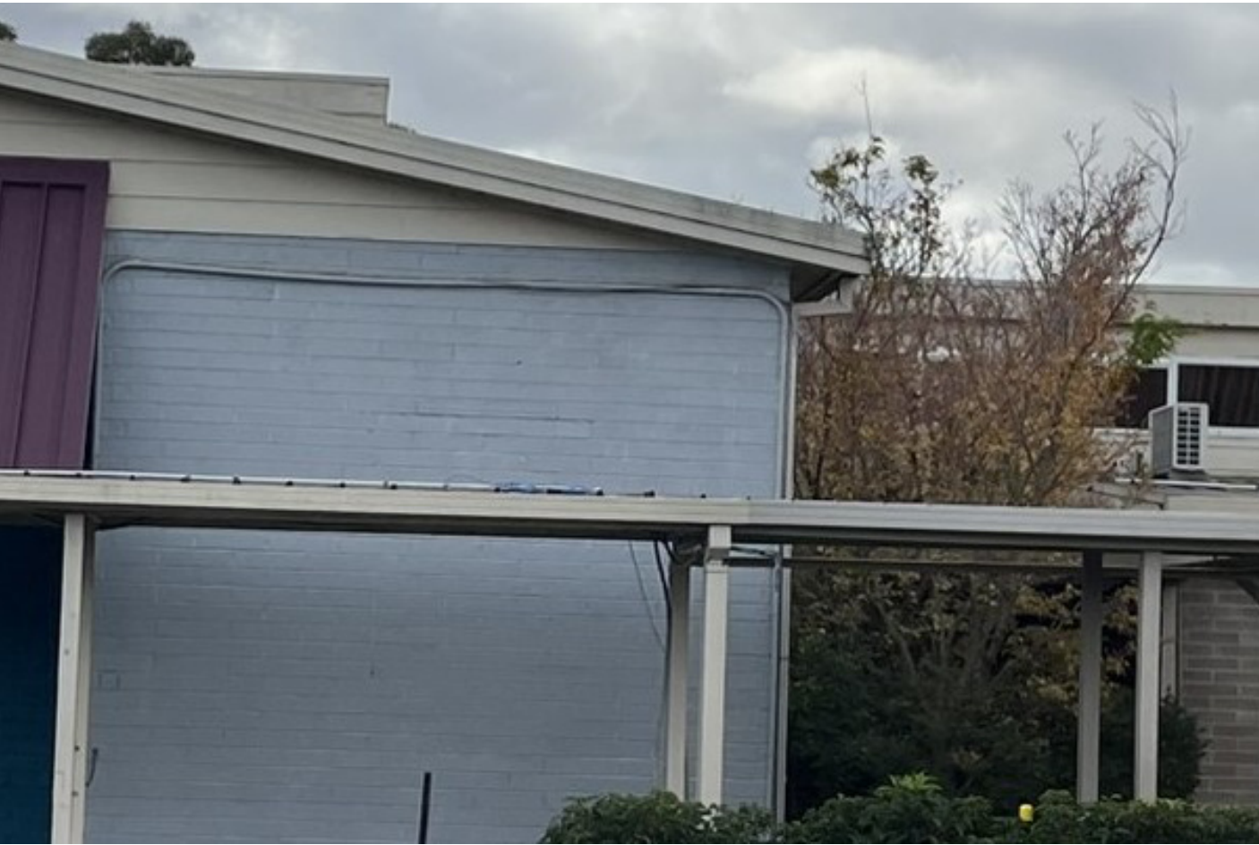
PHOTOGRAPH OF EXISTING EAST SIDE VEGETATION PROPOSED TO BE DEMOLISHED
