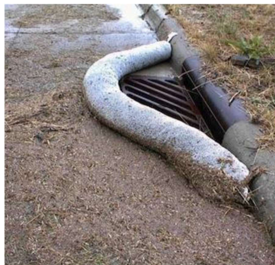
Figure D. Sediment trap (image credit: Delta T Solutions)
