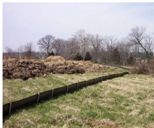
Figure F. Silt Fence (image credit: US EPA, 2008)
