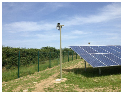
Picture 4 Example CCTV Cameras
