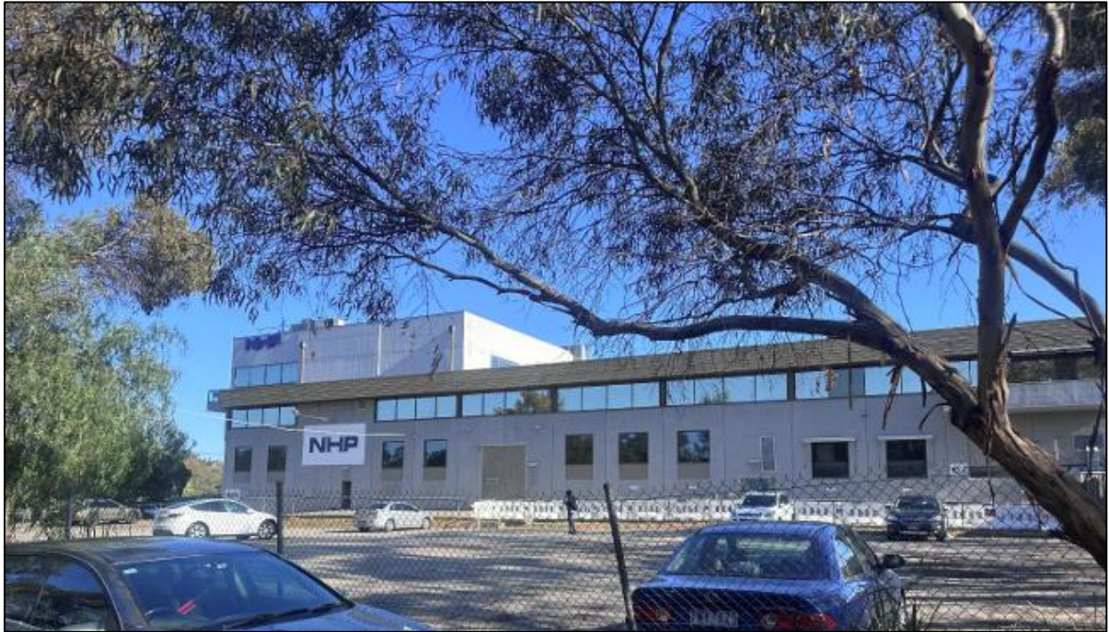
Figure 10: Crown Street frontage (Source: Application)
