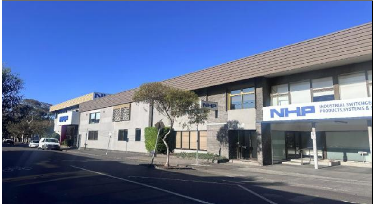
Figure 8: River Street frontage (Source: Application)
