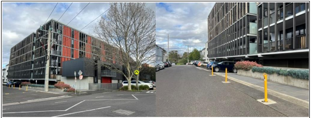
Figure 12: Adjacent building to the south fronting River Street (left) and the private road with carriageway easement (right) (Source: Site visit)
