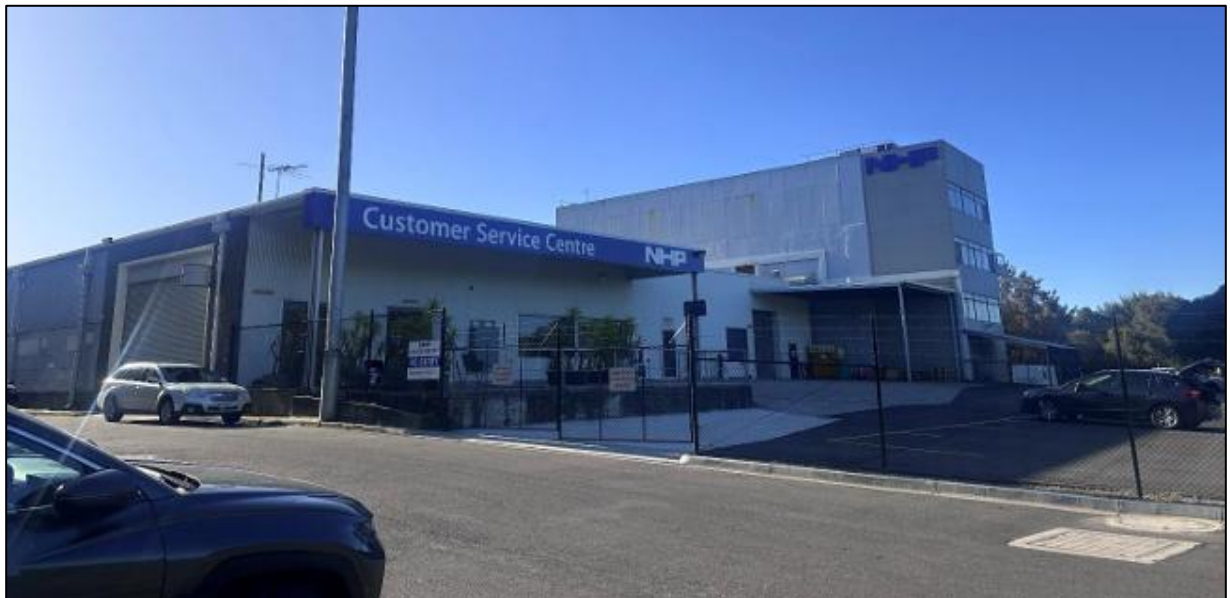
Figure 9: Private Road frontage from the south-east (Source: Application)
