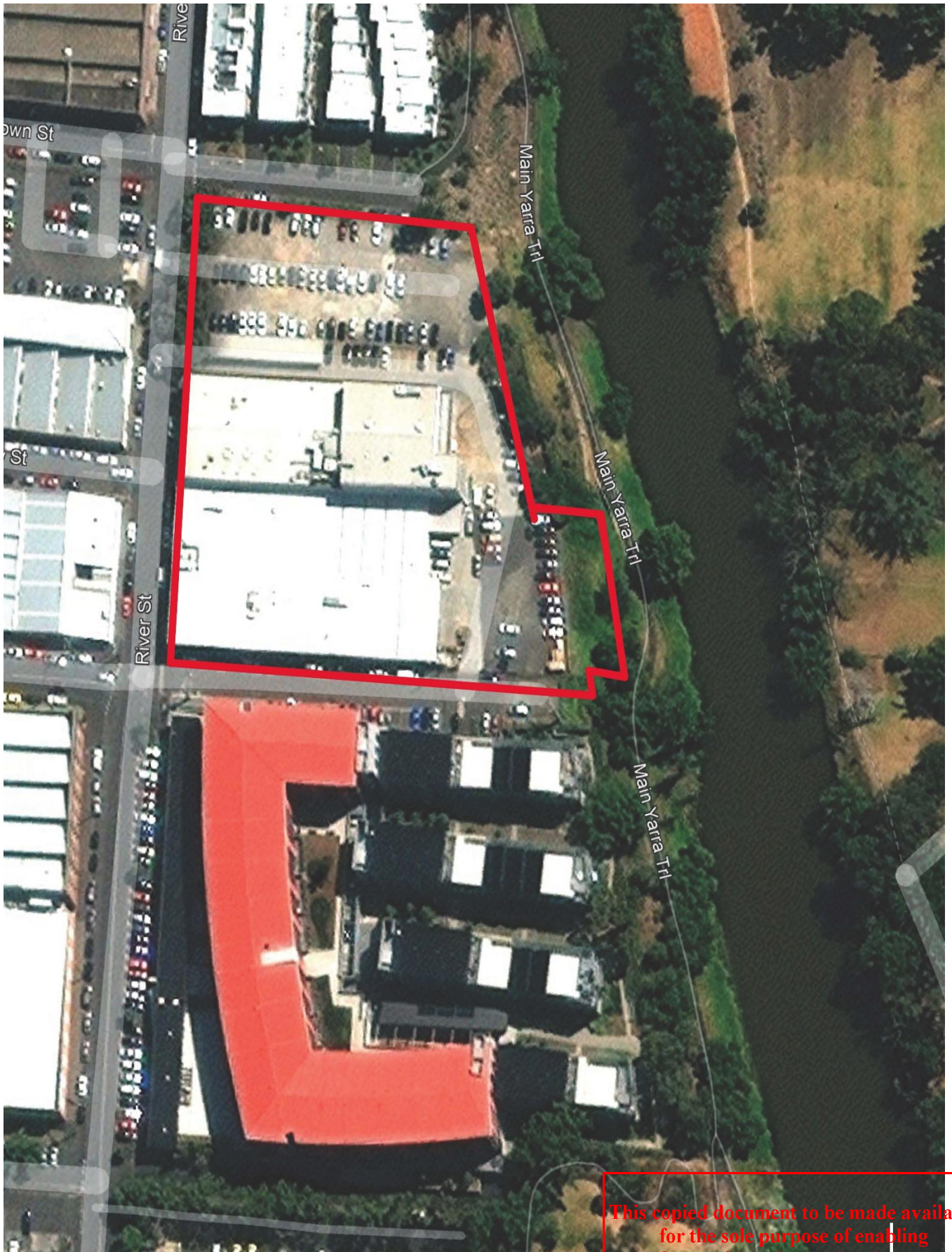
Figure 5 2010 Aerial View of the Activity area (Google Earth)
