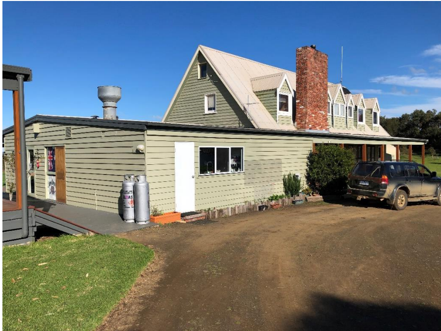
Figure 4 Building Exterior Viewed from Northeast
