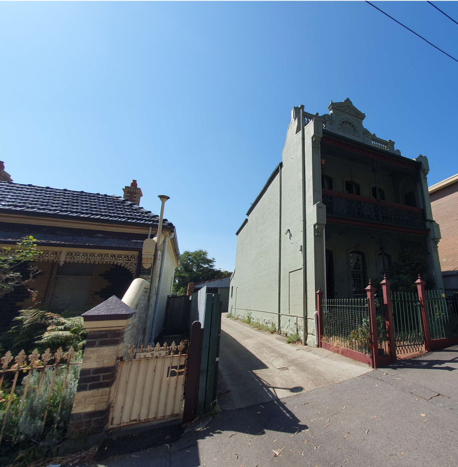
SOUTH WESTERN VIEW OF 46 BROUGHAM STREET, SHOWING WESTERN EXTERNAL WALL
