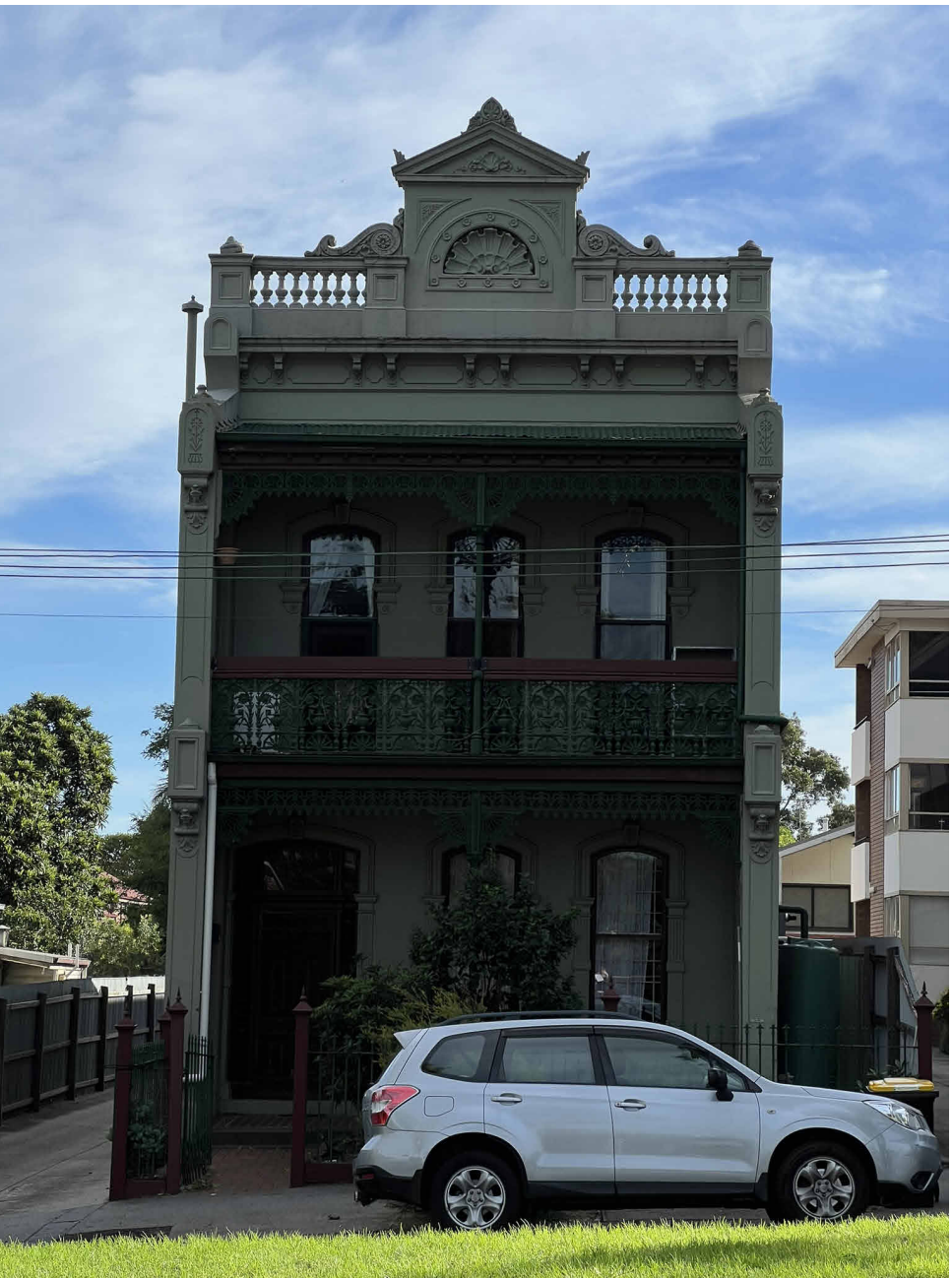
SOUTHERN VIEW OF 46 BROUGHAM STREET, SHOWING MAIN SOUTHERN FRONTAGE.
