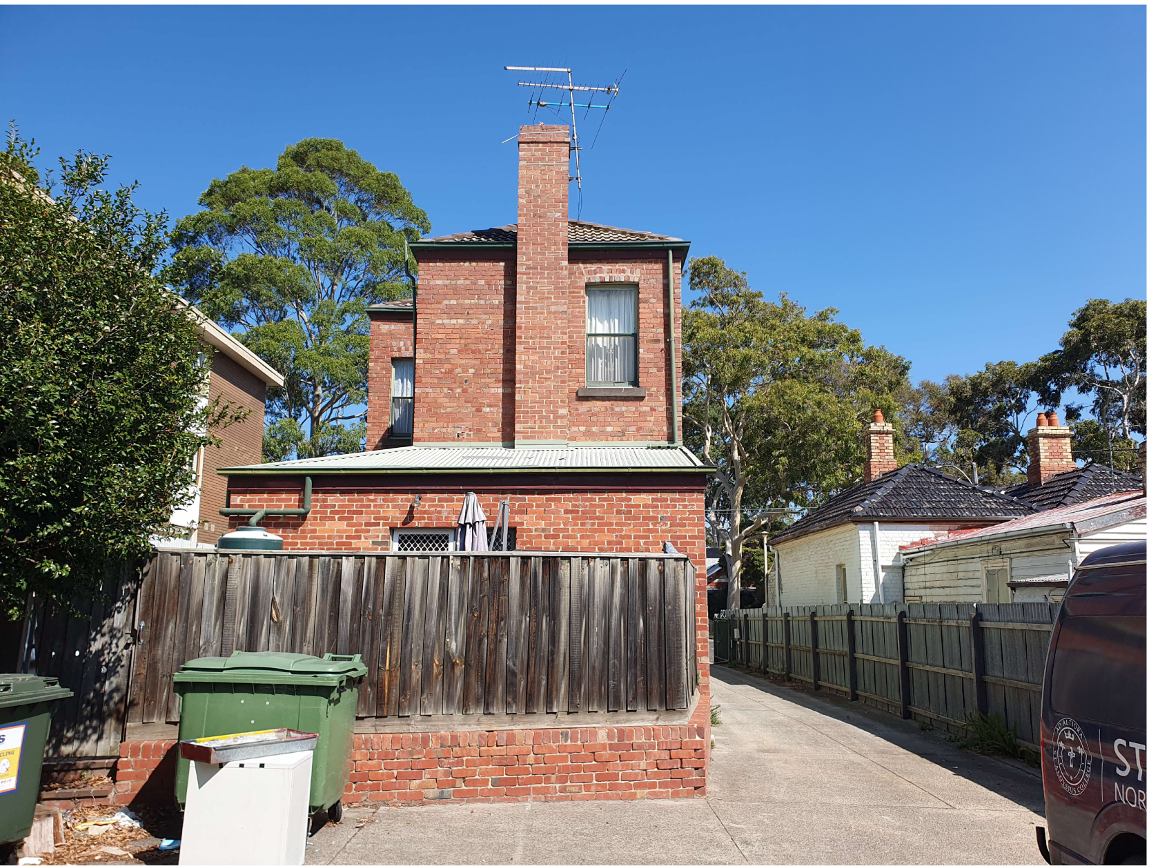
NORTHERN FACADE OF 46 BROUGHAM STREET, SHOWING EXTENT OF EXISTING BUILDING AND GARDEN TO BE DEMOLISHED. SHRUB TO BE REMOVED SHOWN TO LEFT SIDE OF IMAGE.
