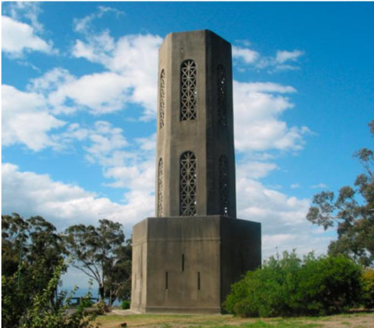
Above: Photograph of former look-out tower (source: Discover Mornington Peninsula).
