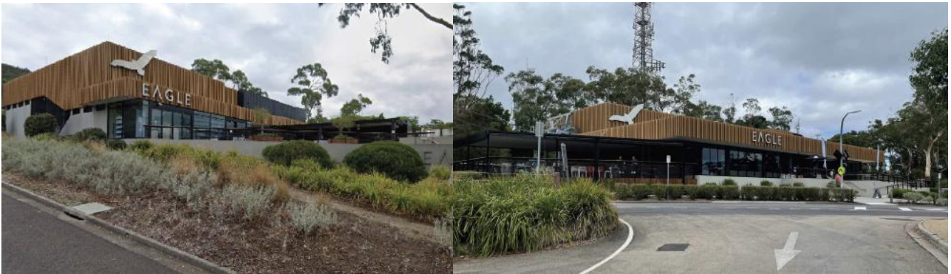
Above: Photograph of existing base station (left) and summit station (right)
