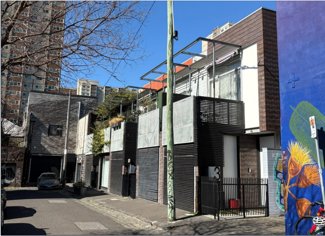
Figure 16. · 3, 5, 7, 9, and 11 Brunswick Place
