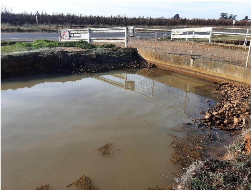
Photo 4 Man-made drainage structure within the study area, 15 August 202
