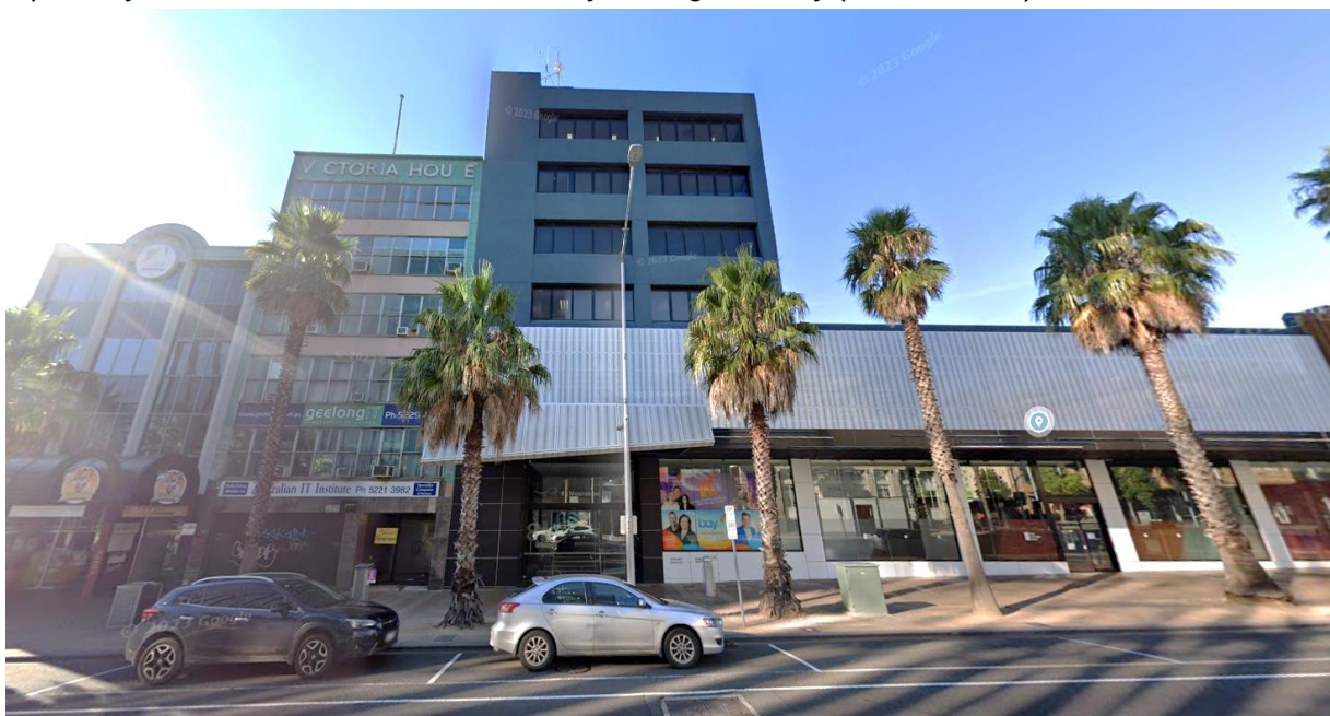
Figure 5. View of 83 Moorabool Street northern frontage
