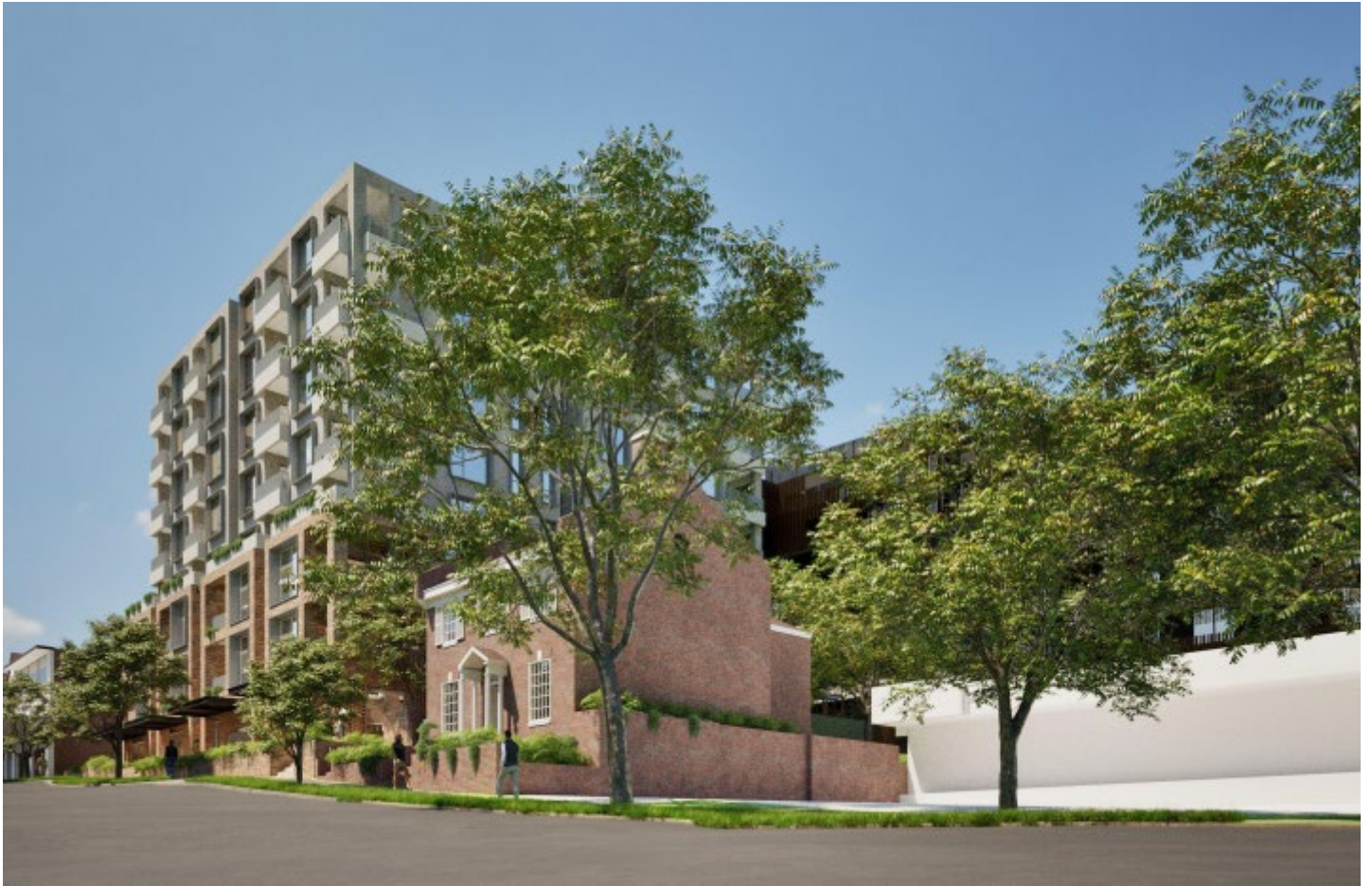
Figure 3: View from Seddon Street looking north west.
