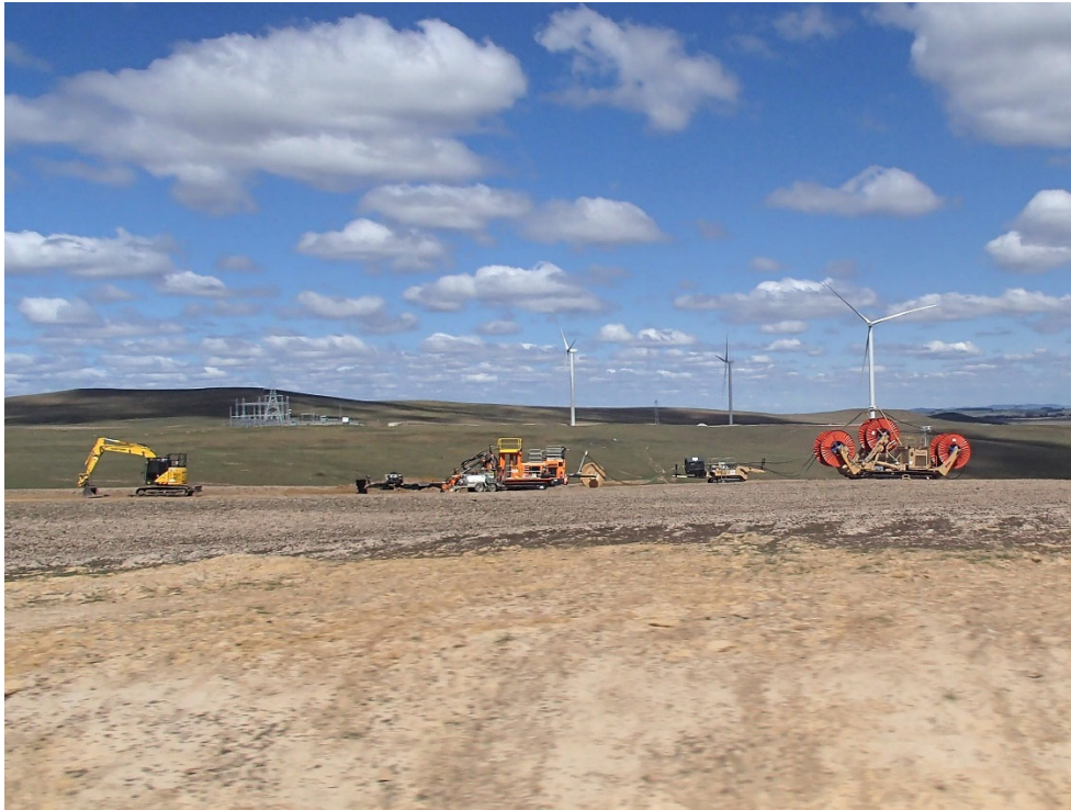
Plate 1 Cable laying equipment
