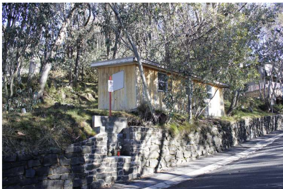
Falls Creek Road
