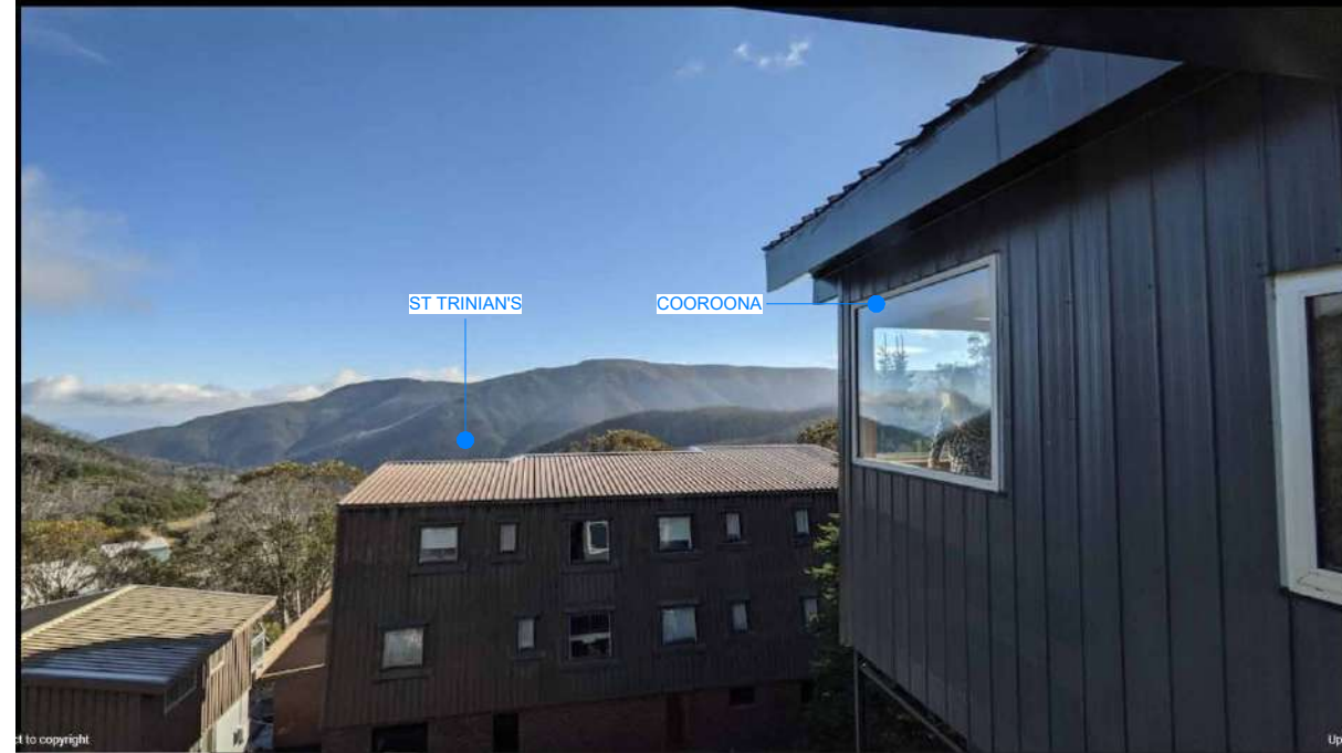
COOROONA PRIMARY VIEW NORTH OVER ST TRINIAN'S
