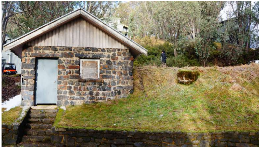
Existing structure on site
