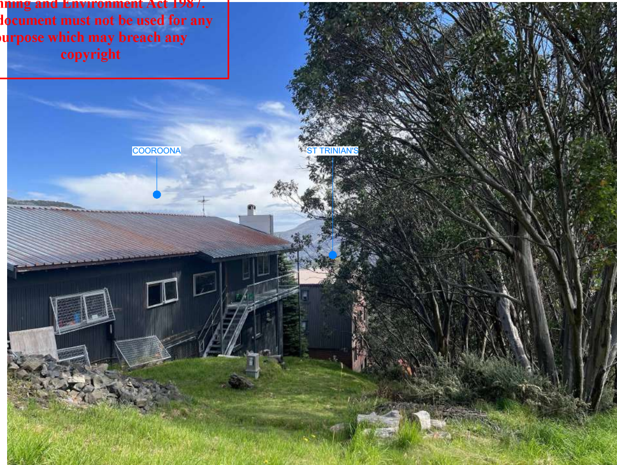
COOROONA VIEW NORTH TOWARDS PRIMARY VIEW. ST TRINIAN'S SITUATED DIRECTLY IN FRONT. TALL TREES TO THE EAST.
