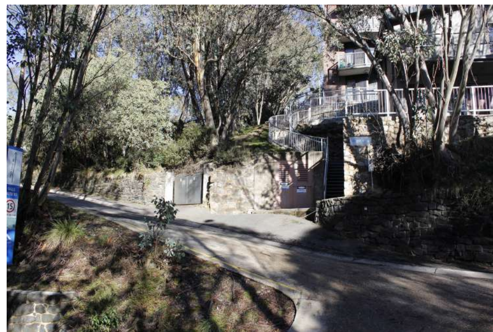
Lot 4b substation
