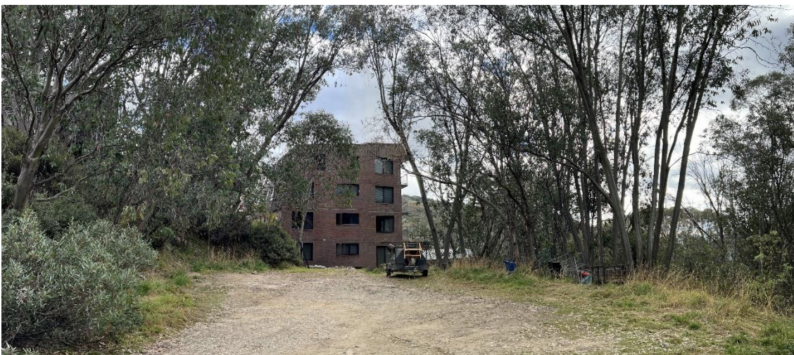
View west across subject land with four storey building (St Trinians) in background
