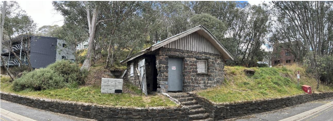
Image of the existing building viewed from Christie Street
