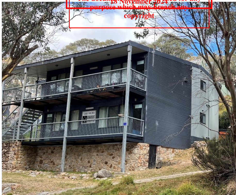
View north side of Southern Cross Apartments
