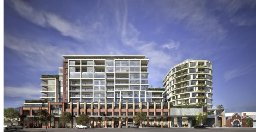
Picture 12 Western Interface Render – Demonstrating consistent rhythm of street wall and podium
