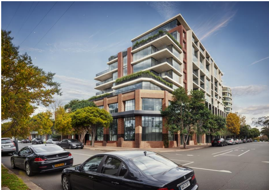
Picture 13 – Sinclair and Selwyn Interface – demonstrating recession above podium to residential interfaces
