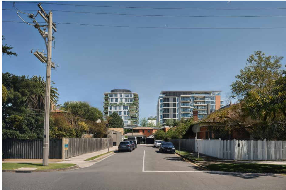
Picture 15 Eastern site perspective - demonstrating visibility from May Street an St Georges Road
