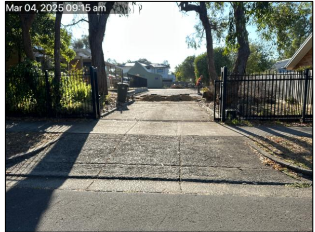
Photo 2. The western site entrance and area of proposed ramp to basement.
