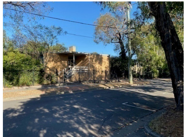
View six – Main pedestrian entry to existing building (Witt Street)
