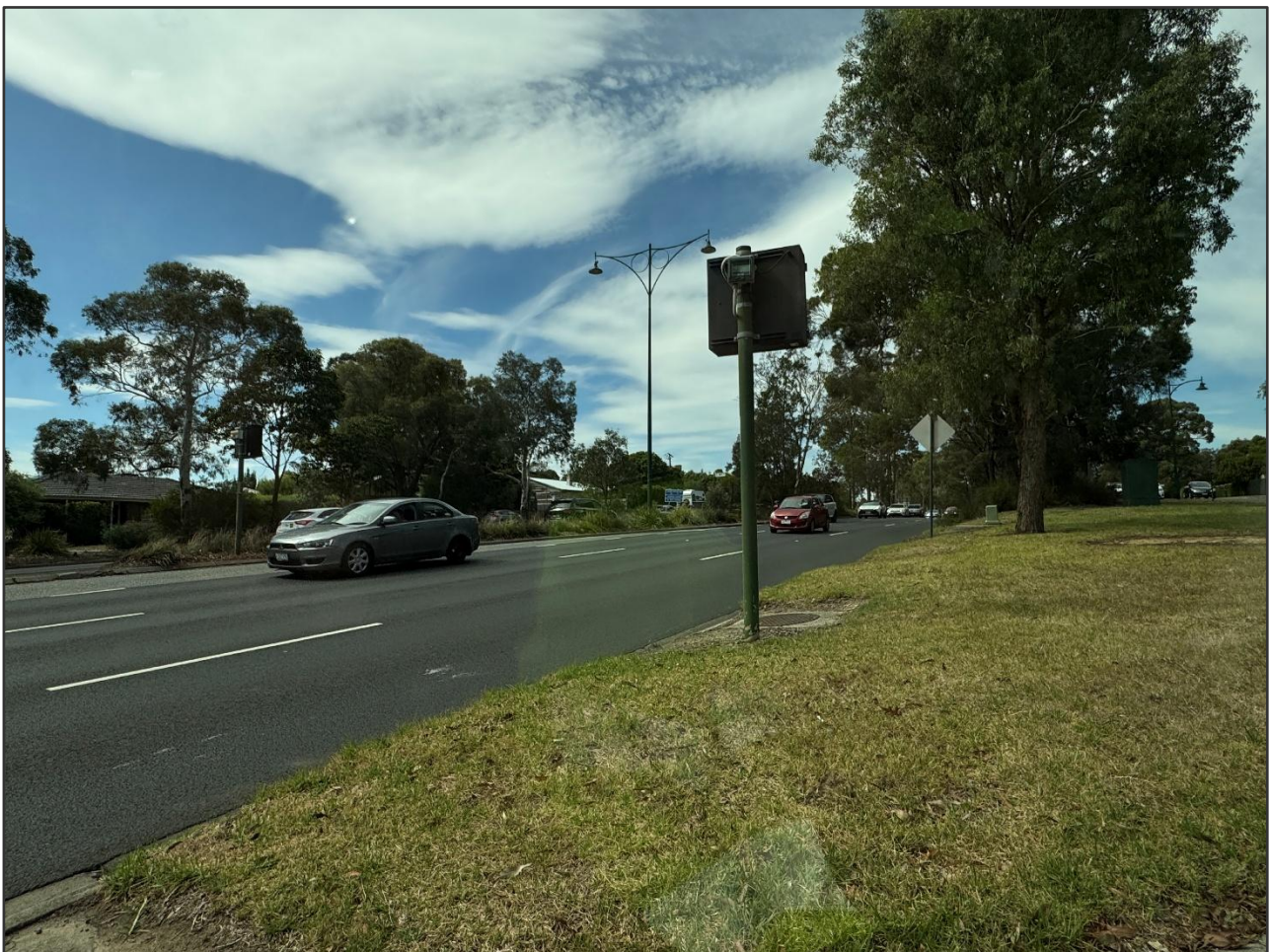
Figure 7 Whitehorse Road, looking east from the Service Road
