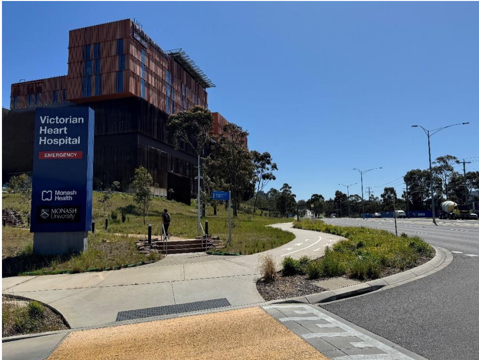
Figure 11: Signage on adjacent Victorian Heart Hospital, Blackburn Road (pedestrian for scale)
