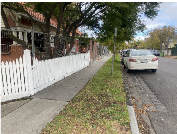
Figure 3-13. Bluestone kerb and drain at 101-103 Droop Street (The Crescent), facing southwest
