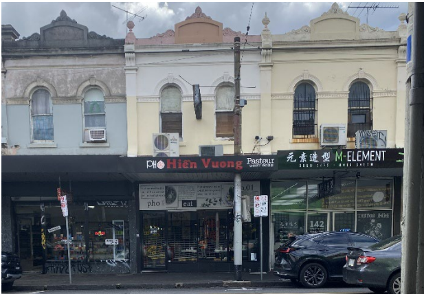
Figure 3-22. 144 Hopkins Street with overhead pole through the awning, facing north
