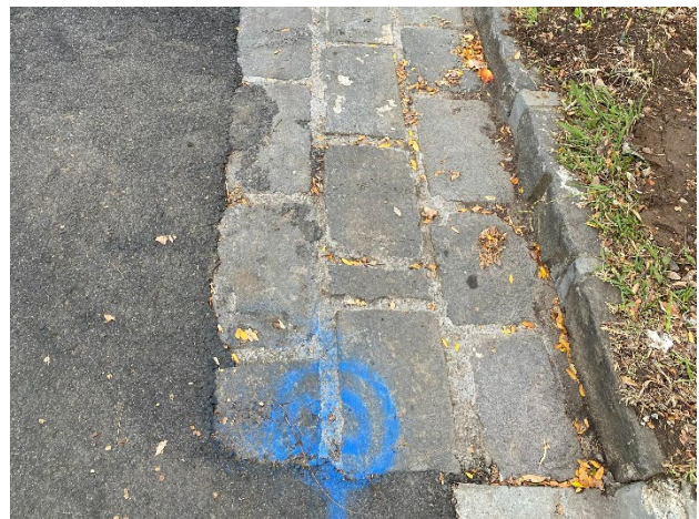
Figure 3-14. Closeup of bluestone kerb and drain at 105 Droop Street (The Crescent), facing southwest
