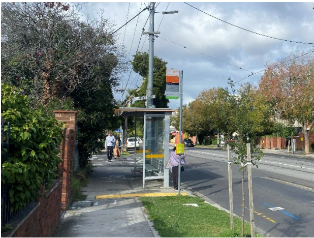
Figure 3-11. Existing tram stop and shelter on Droop Street, facing southeast
