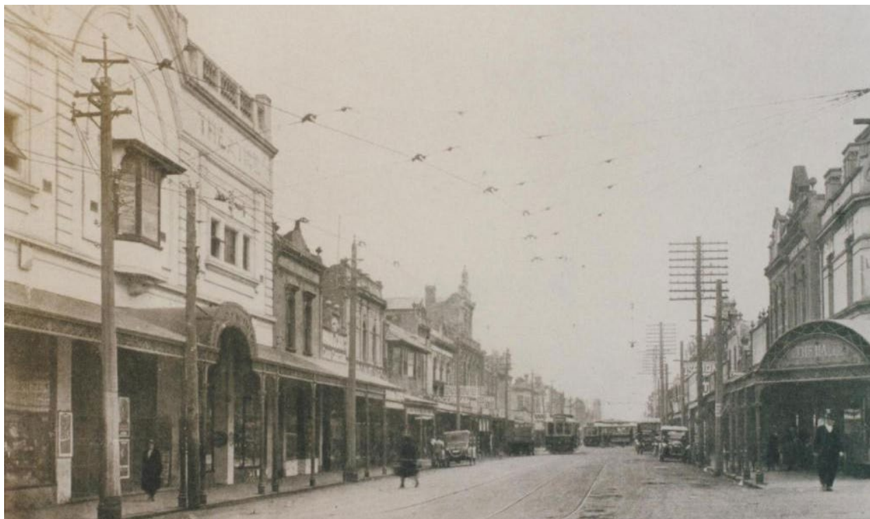
Figure 3-15. Tramlines running between the shops with post-supported verandahs along Hopkins Street in 1924, facing west towards Droop Street (John Young Collection 1924)
