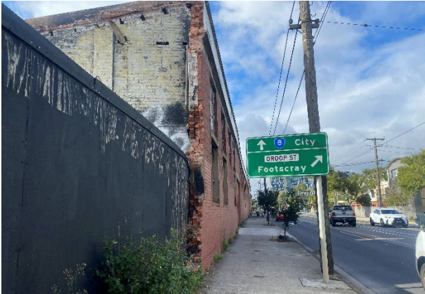
Figure 4-8. Part of Kinnears Ropeworks Footscray, facing east
