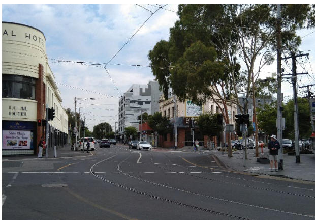
Figure 3-16. Within the Footscray Commercial Heritage Area (Maribyrnong HO3) precinct, facing northwest towards Droop Street
