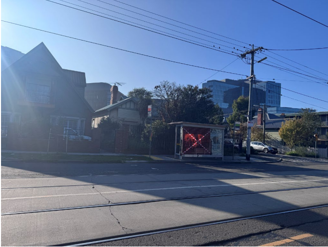
Photo 1: Existing tram stop shelter on the eastern side of Droop Street.
