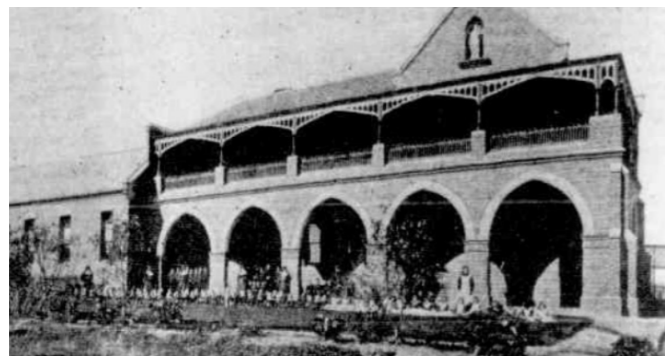
Original facade, as seen on photo taken on 16 September 1901
