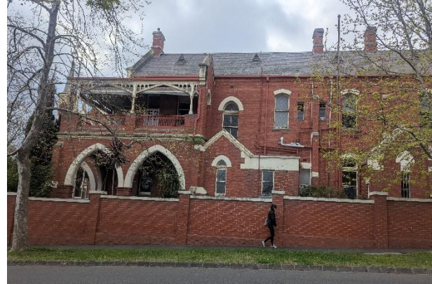
Figure 11 Western elevation of c.1889 main building showing the original verandah within pointed arches and balcony on the first floor
