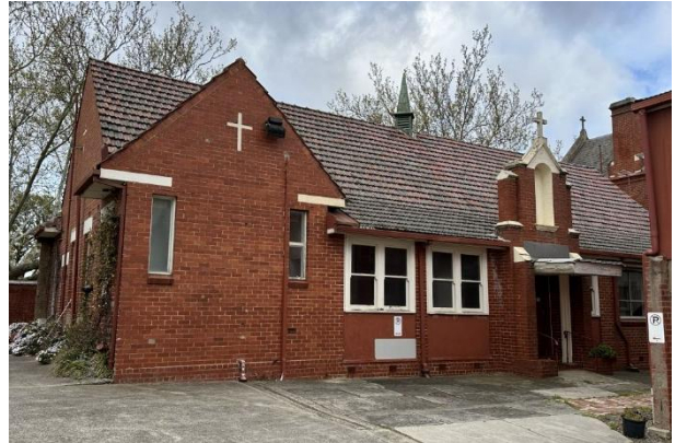
Figure 17 Northern elevation of the infirmary as viewed from within the site
