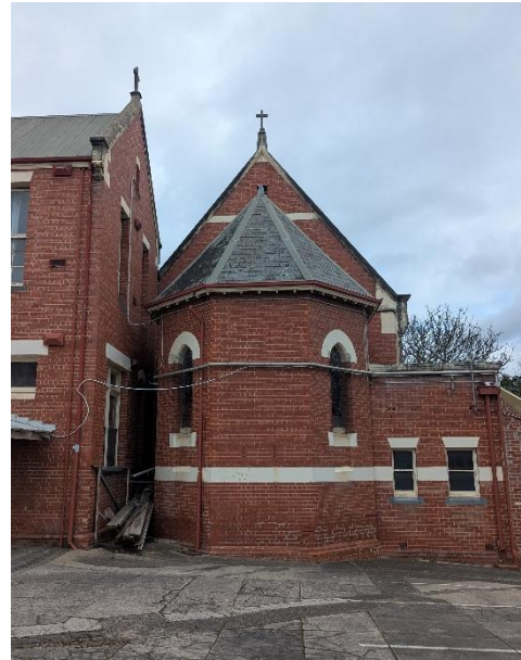
Figure 15 Eastern (rear) elevation of the Chapel showing the northern entrance bay
