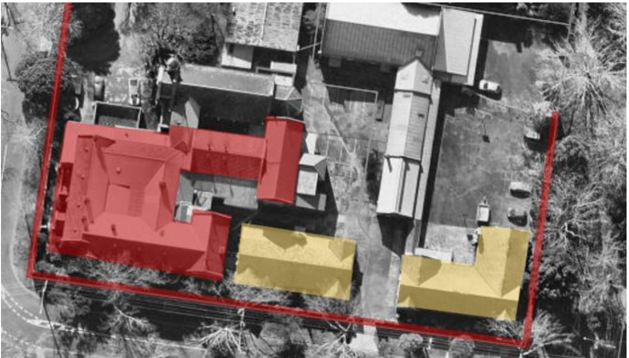
Figure 26 Elements of primary significance indicated in red; contributory elements in yellow: note the significance perimeter wall extends to the north along Middlesex Road Source: Lovell Chen (Nearmap as base)
