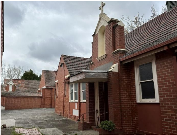
Figure 18 Northern elevation of the infirmary showing the enclosed verandah
