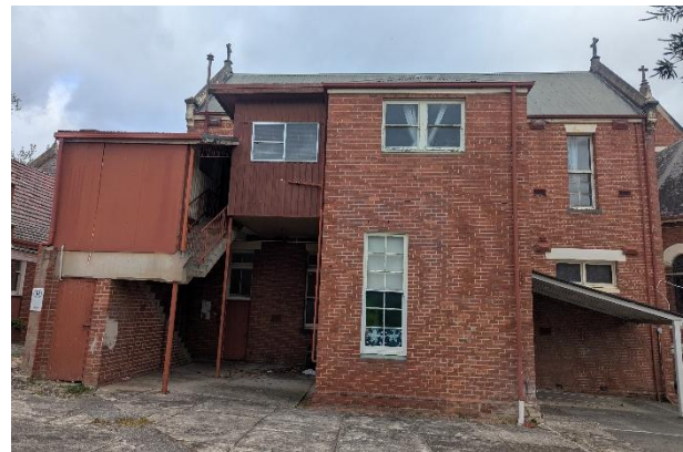
Figure 13 Eastern elevation of the 1907 addition showing intrusive later additions
