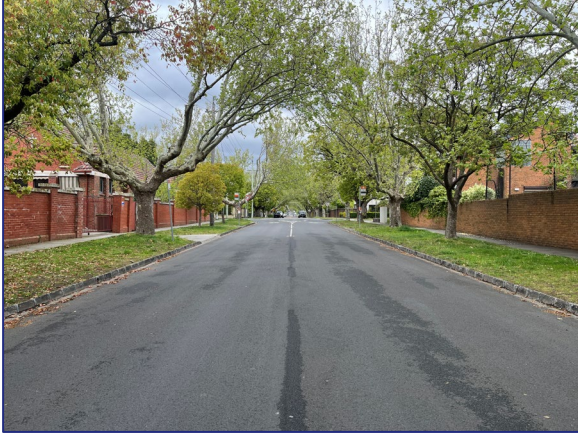
Figure 6: Kent Road – view east
